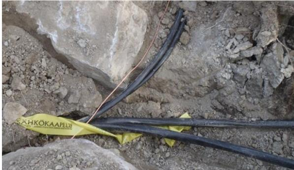
Figure 2. *Sharp rocks are left near the cables, contrary to installation guides.*
